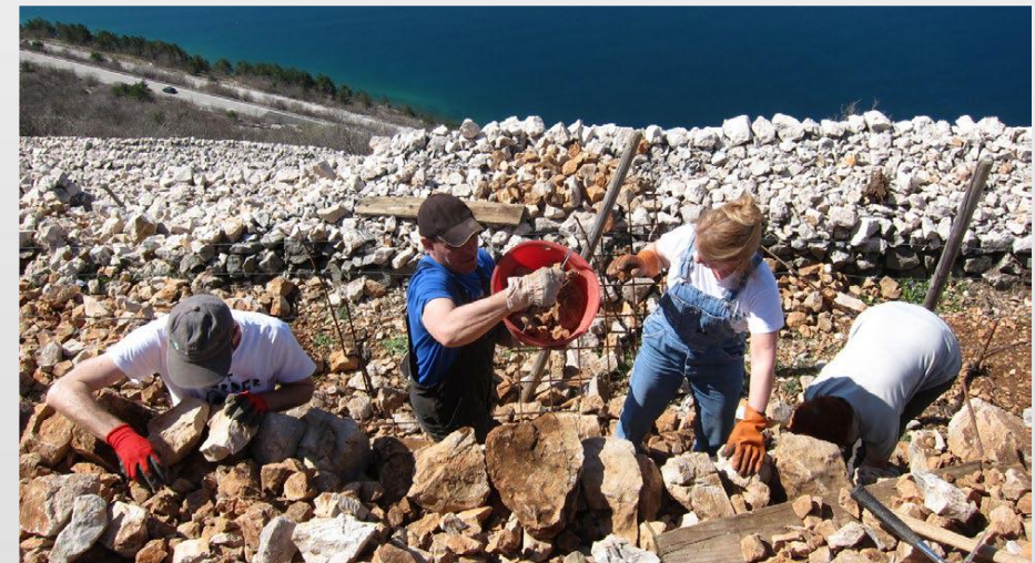
Repairing dry stone terraces of the Takala vineyard, the first protected dry stone landscape in Takala, Croatia, 2018. Photographer: © Filip Šrajer, Dragodid
