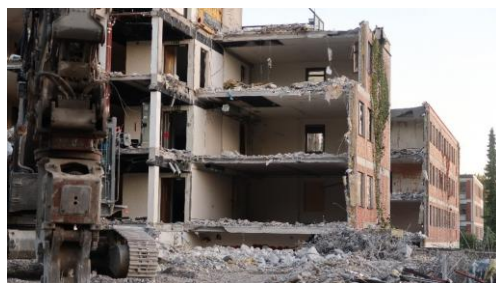
Demolition of buildings
